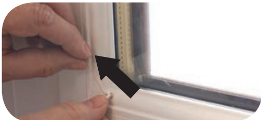
11. Holding button, pull cord tight to secure.
