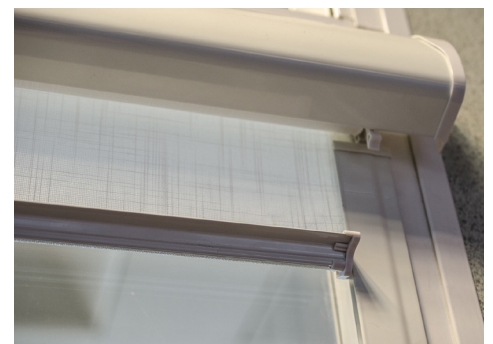
11. On opposite side, tilt bottombar to open position and slide side extrusion over bottombar end cap and fabric ensuring both are within the fabric channel on the side extrusion.
