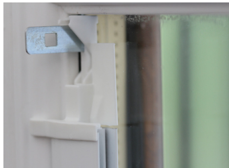
8. Apply pressure to click home the profile top end cap.
