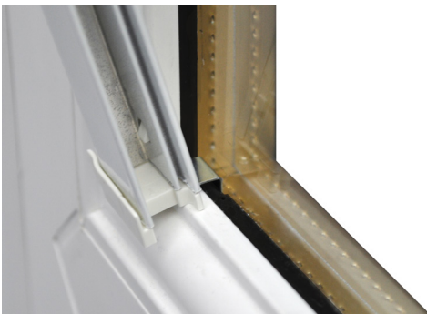
7. Locate the profile bottom end cap over the bottom bracket.
