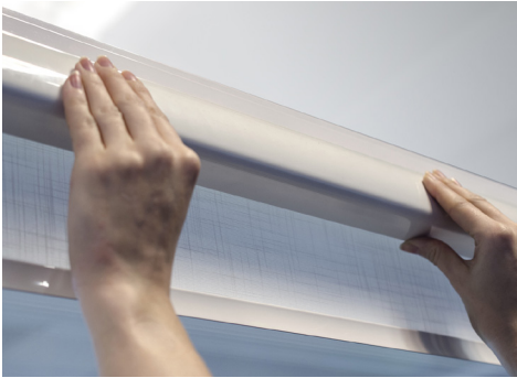
10. The blind can now be pushed fully home onto brackets.
