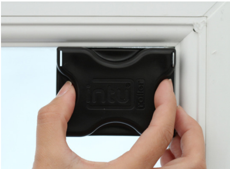
4. Insert the bracket behind the rubber seal until the tool edge touches the bead at both top & side. Repeat for other side.
