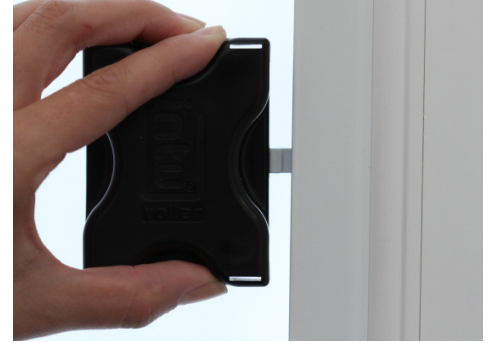
10. Position relevant number of recommended side extrusion clips according to the drop of the blind. Push home the extrusion clips with fitting tool.
