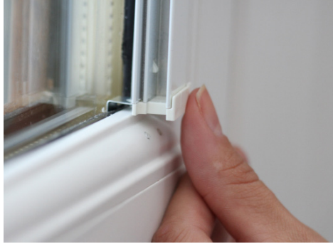
10. Engage the side extrusion bottom bracket into the bottom corner fixing bracket.
