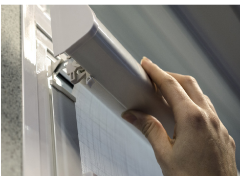
10. Slide the headrail onto top corner brackets on both sides. N.B Do not push blind fully home onto brackets
