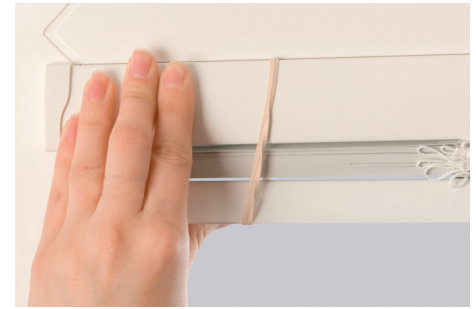
15. Ensure headrail is correctly aligned and firmly press home. Snip off rubber bands and lower the slats fully.
