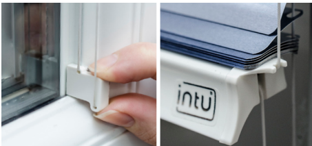
16. With cords at bottom of bracket, slide onto clip. Repeat both sides. Ensure the front cord sits within the notch of the bottombar endcap.
