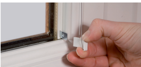
16. With cord at bottom of bracket, slide onto clip. Repeat both sides.
