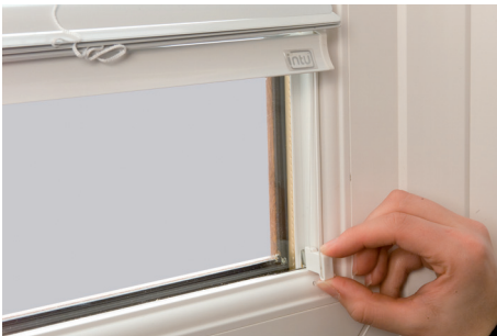
16. With cord at bottom of bracket, slide onto clip. Repeat both sides.
